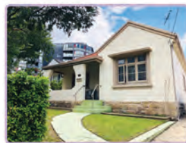
St Andrews House Gladesville
