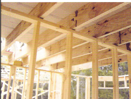
Pine structural framing, LVL beams
