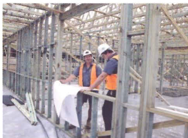
Pine termite treated framing
