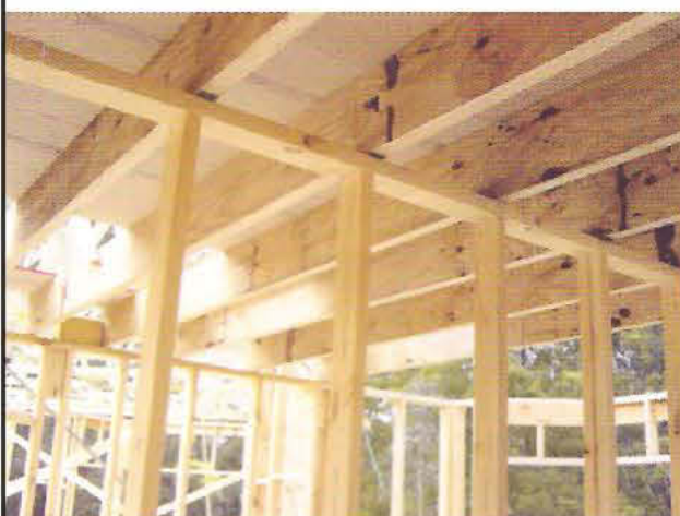
Pine structural framing, LVL beams
