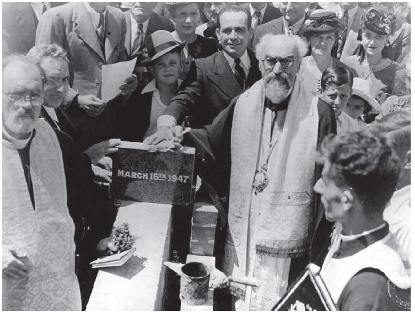
A Greek Orthodox priest applies mortar to the foundation stone of St.Theodore's Greek Orthodox Church in Townsville on 16 March, 1947
