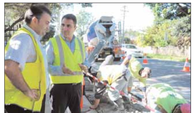
Burwood Mayor John Faker inspects the second phase of the works on Queen Street.
