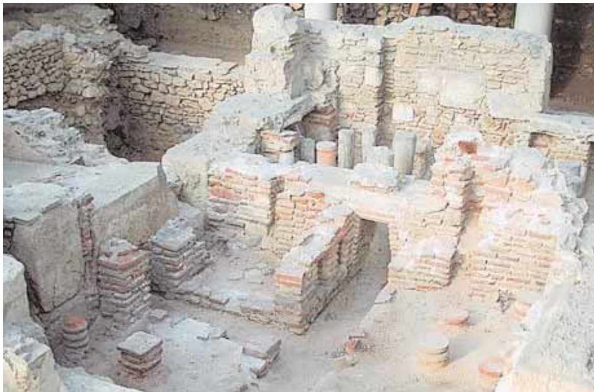
Construction of an air vent near Syntagma revealed a well-preserved Roman bath
