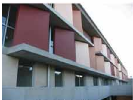
Rear of the building
